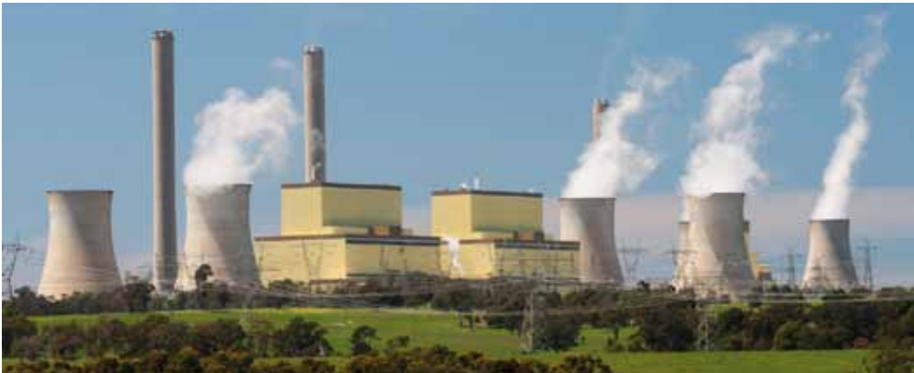
Coal Fired Power Station
